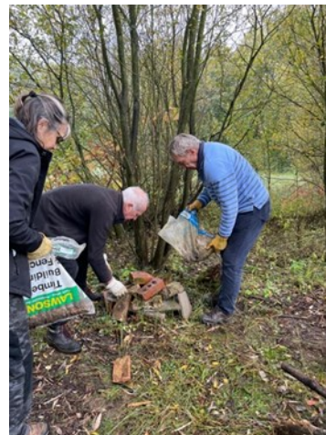
The hibernaculum in construction and complete.
