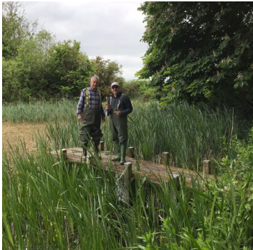
Jetty repairs Picture by Cathy Eckett
